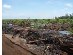
Soils dug out from the drainage canal
